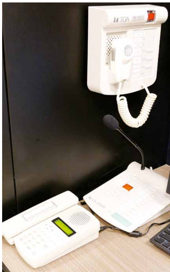
Announcements in the FCC can be made from the RM-200SA, IP and RM-200SF microphones
