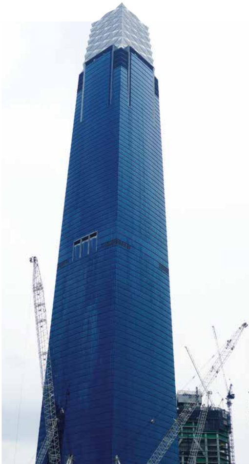
Exchange 106 has risen majestically above the TRX site
