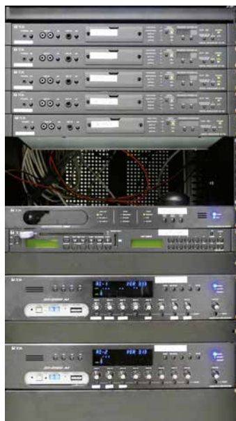
SX2000SM control rack in the FCC
